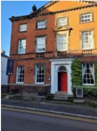
The Bank House Hotel Church Street, Uttoxeter ST14 8AG
