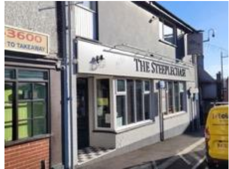
The Steeplechase 58 Bridge Street, Uttoxeter ST14 8AP
