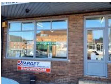
Target Windows 1 Smithfield Road, Uttoxeter, ST14 7LG
