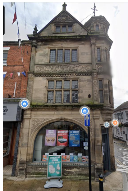
Mill Outlet The Old Warehouse, Market Street, Uttoxeter ST14 8JA
