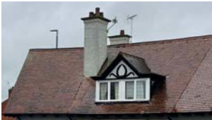
Red pantile and chimney stacks
