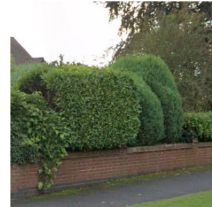
Low brick wall and tall vegetation
