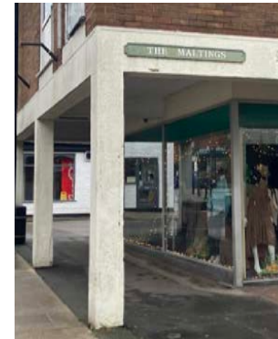
Concrete columns for colonnade at The Maltings
