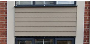
Weatherboard cladding between windows as bay frontage
