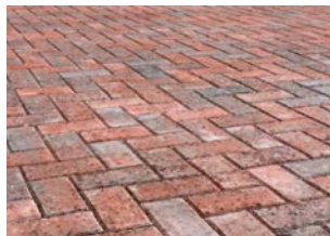
Red brick block paving in residential streets
