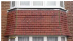
Shingle tiles on bay windows
