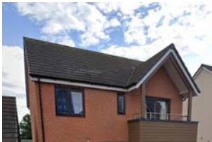
Roof overhangs on balconies
