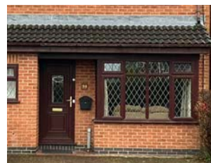
Skirt roof entrance
