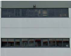
Cladding panels and strip windows
