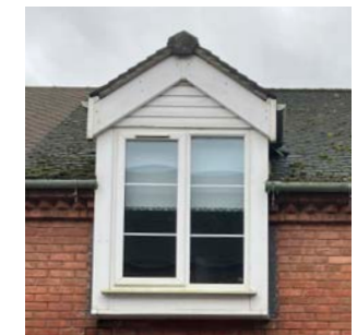
Dormer casement windows and gable end
