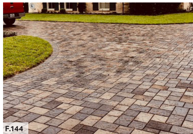
Figure 144: A good example of permeable paver (Source: https://www.paverconnection.com/testimonial/hedwig-village-permeable-drive-way-and-patio-upgrade/ )
