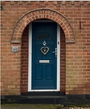
Recessed doorway and arched entrance
