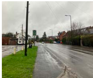
Green verges on primary roads
