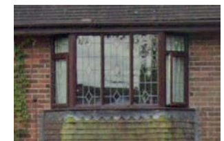
Brown timber bay windows
