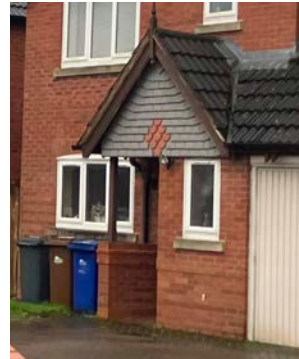
Gable front porch with fascia
