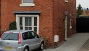
Side entrance with no porch
