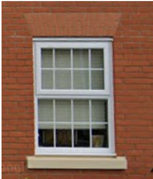
Sash style window with mullions
