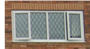
Casement window with diamond muntins
