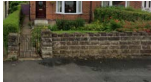
Low limestone/brick walls
