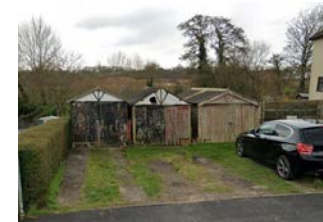
Standalone garages in disrepair and underused
