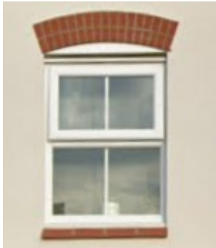
Sash style window with curved brick lintel
