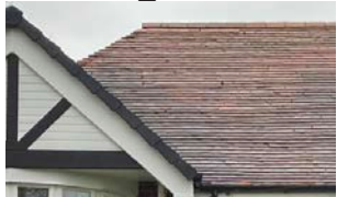
Timber fascia roof and red pantiles
