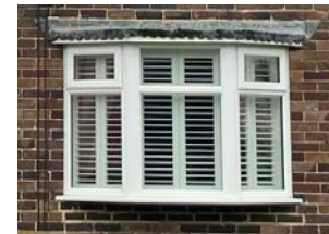
Bay fronted windows
