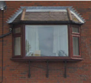
Oriel bay window with supporting brackets
