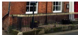
Metal fencing along Church St
