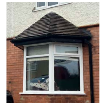
Bay windows with hip roof and uPVC window
