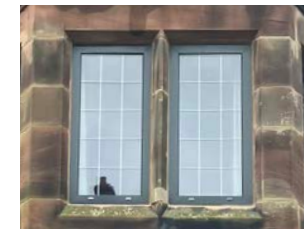
Limestone windows and lintels with mullions
