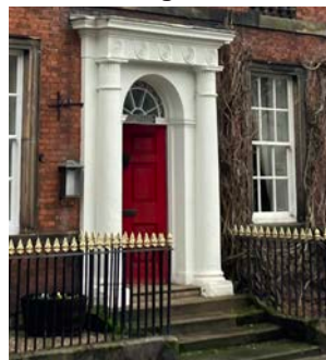
18th century frieze, engaged piers and arch
