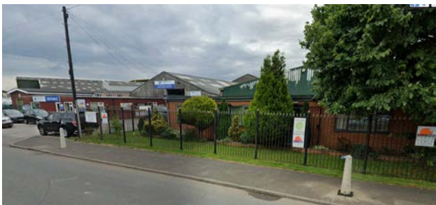
Tall metal fences, bollards and trees create a visual and physical barrier between the street and the property
