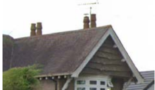
Concrete tile, timberboard/ batten eaves
