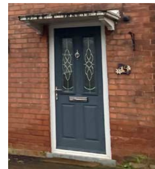
Concrete flat roof porch with uPVC door
