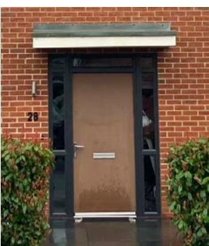
Flat roof with timber door
