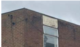
Parapet roof and coping stones at The Maltings
